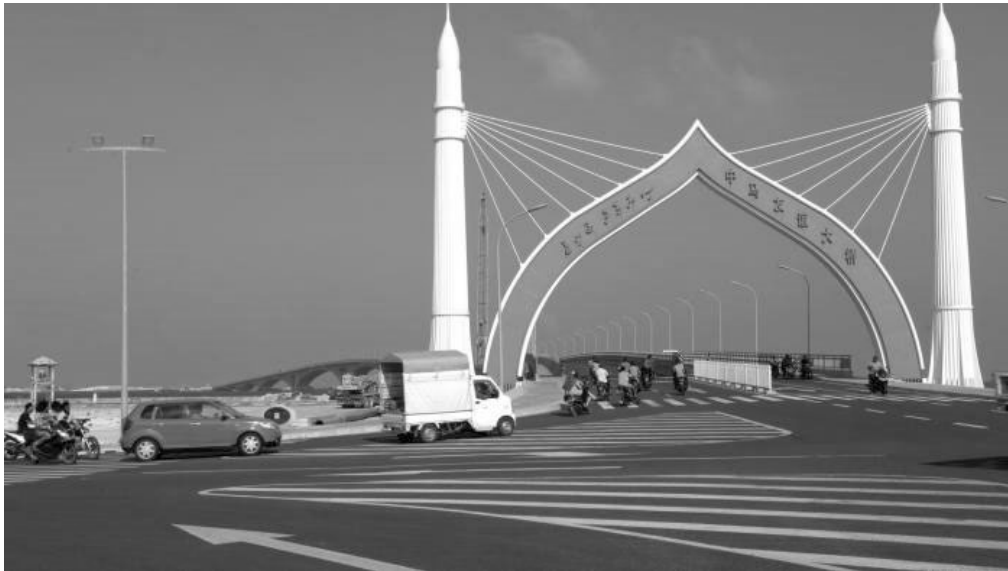
Figure 3: Maldives-China Friendship Bridge linking Capital Malé to International Airport
